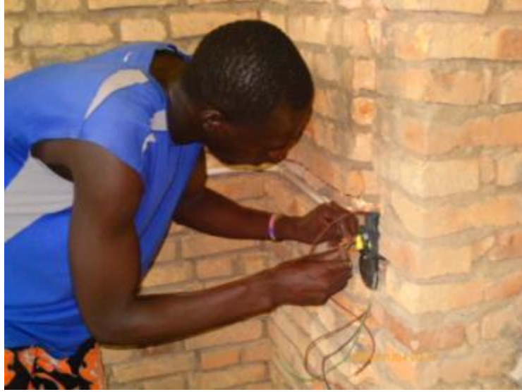
Me wiring a junction box
